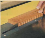
Separate the molded edge. Once the profile has been completed, rip off the edge of the board on a tablesaw.
